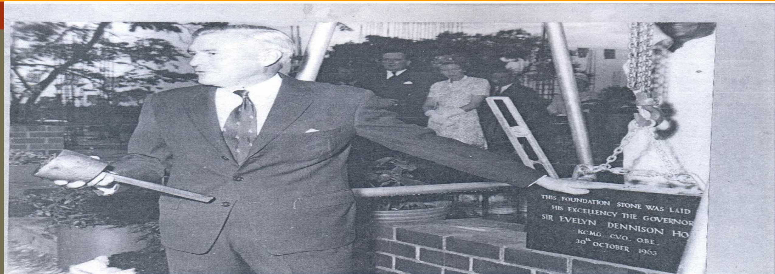
Sir Evelyn Hone - Governor of the then, Northern Rhodesia laying the foundation stone for NIPA (then Staff Training College) on 30 th October, 1963
