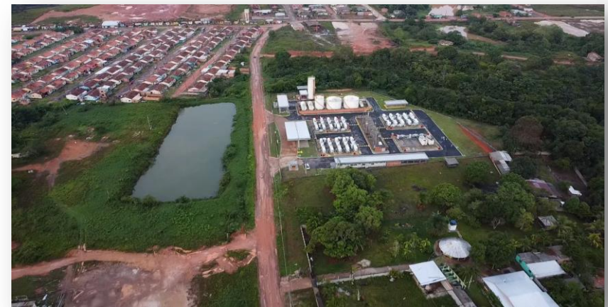
Diesel oil thermal power plant (Castanho II – 20 MW)
