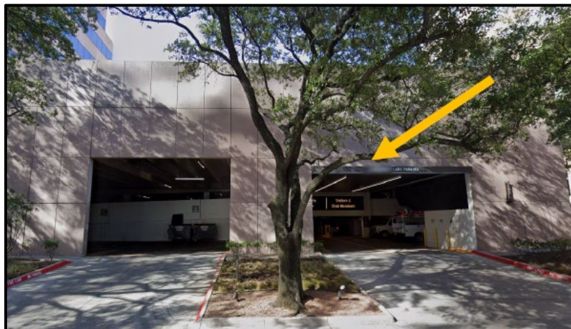
Parking Garage Entrance
